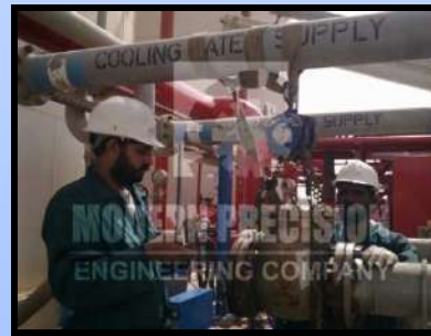
Valve Removal & Installation
